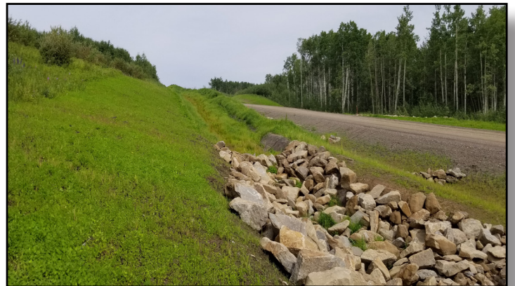
Permanent TRMs can be used to stabilize channels alongside project roadways.
