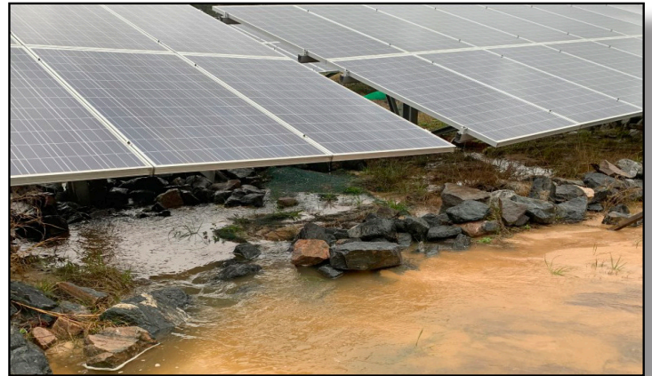
Solar farms can see issues with drainage in and around the installed panels, creating issues with sediment movements.
