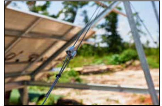
Falcon LockGrip tensioners can be used to tension cable braces on solar rack installation. Whether in a cross or whiplash configuration, the LG-3 can increase the total working load.
